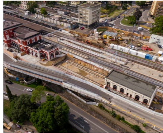
Lugano-Besso underpass construction site.
