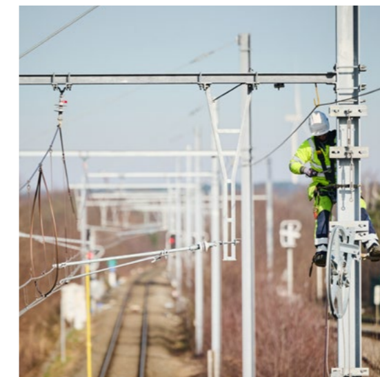
Electrification works between Genk-Goederen and Bilzen (L21C)
