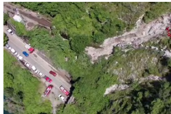
Top view of the landslide
