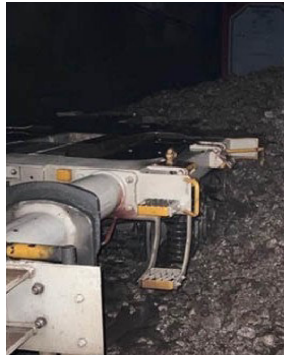
Freight train derailed inside the Laveno tunnel
