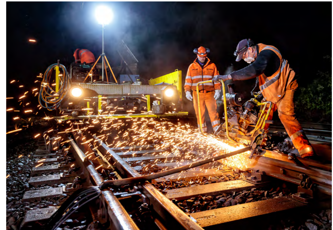
Track work by DB Netz AG in Koblenz.
