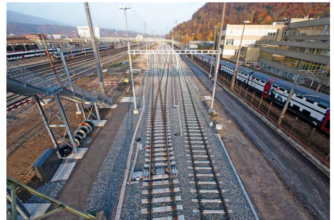
New tracks laid in Olten East (Switzerland).
