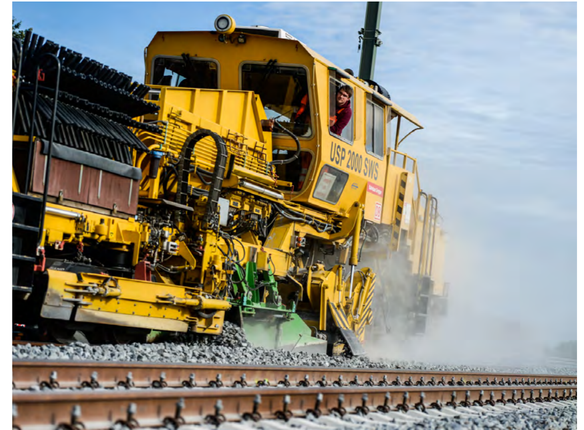
Ballast leveller in operation on the German network.
