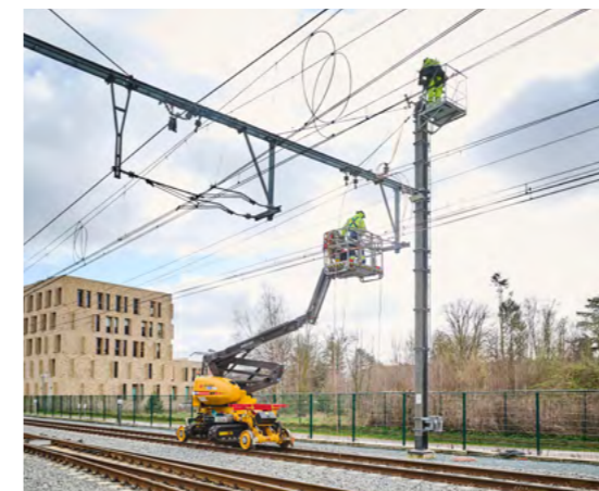
Electrification works on the line between Mol and Hamont (L19).
