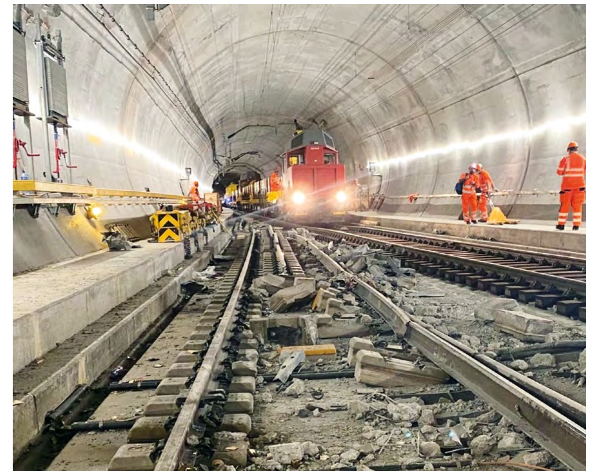
Clean-up work in the eastern tube of the Gotthard tunnel.
