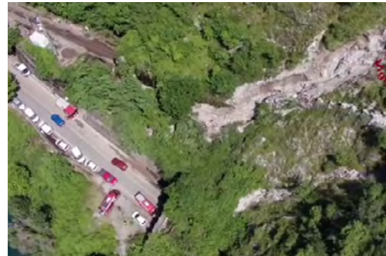
Top view of the landslide
