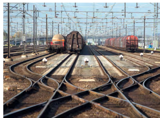
Railyard in the Netherlands.
